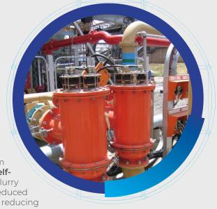
**Kleerflo** Filters are uniquely suited to the tough conditions experienced on mines. They are low in maintenance, durable and efficient in removal of suspended solids. They are self-cleaning.
