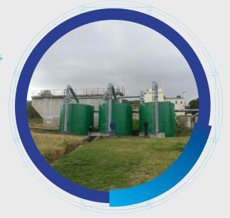
They selected 3 x **AGF42S** (97m<sup>3</sup>/h per unit @ 7m/h) **autonomous, mechanical rapid gravity sand filters.** Since commissioning in 2004 the AGF filters have consistently produced high quality filtrate and fulfilled the requirements that the process / design engineers set.
