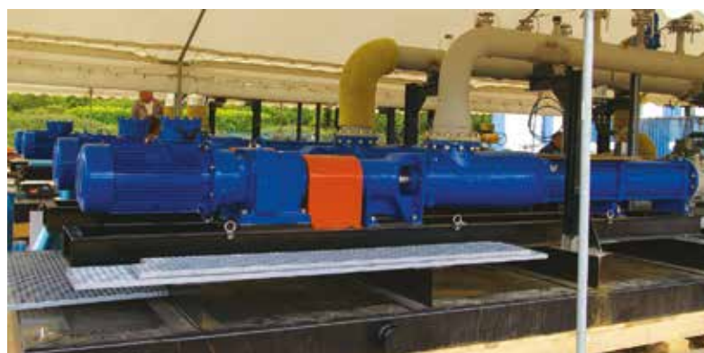
Progressive Cavity Pump
